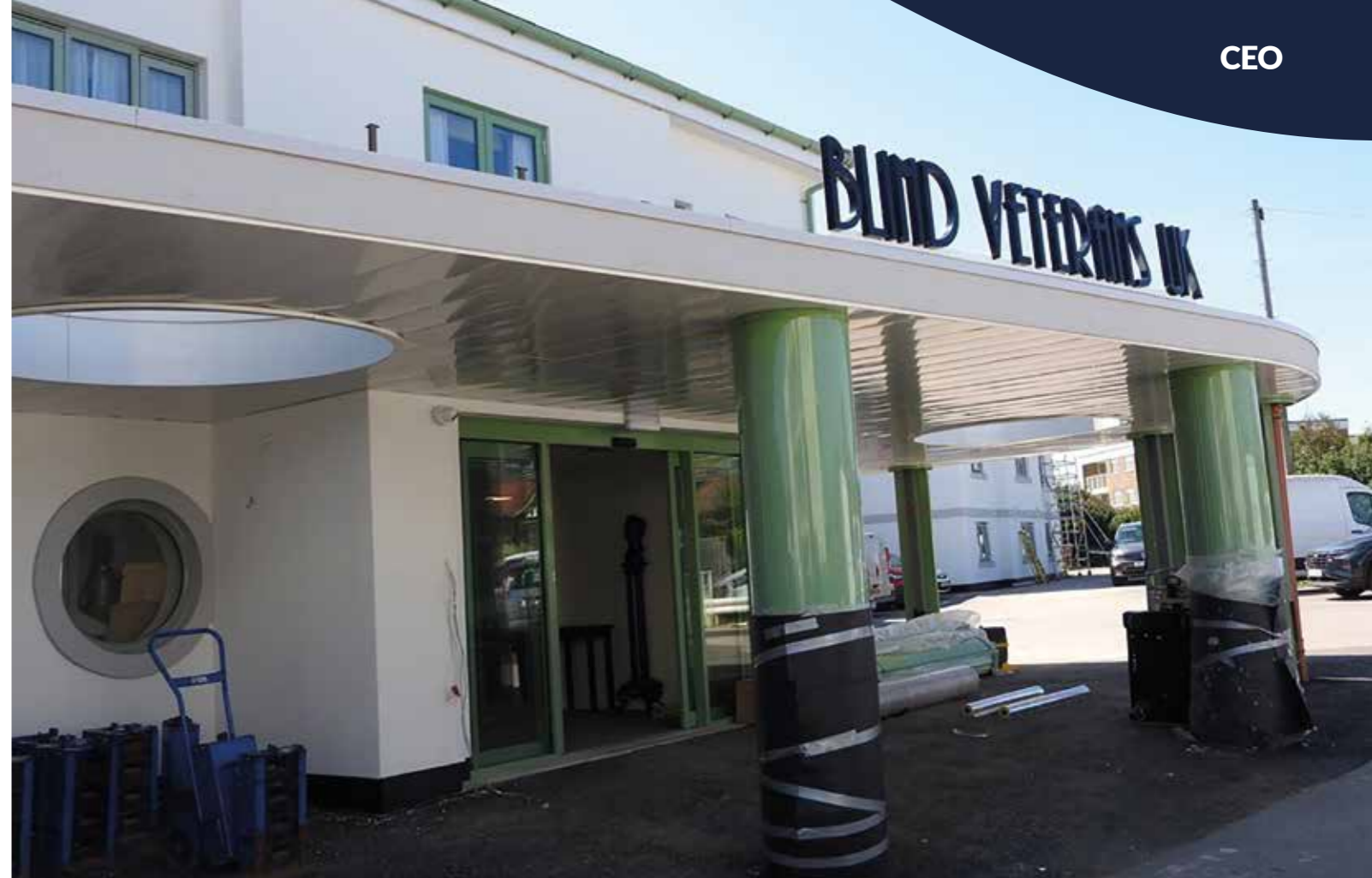
Caption: The front entrance of the Rustington Centre
